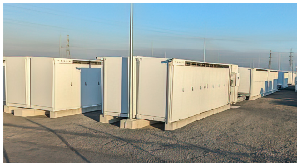
The Victorian Big Battery near Geelong comprises 106 of these Tesla BESS units [R. Thiele, FBICRC].
