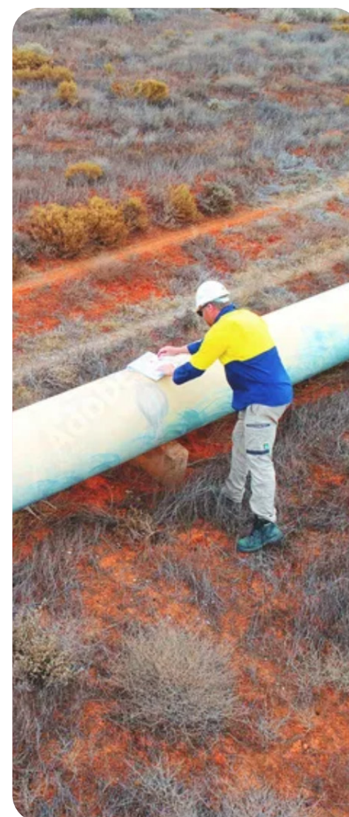
Figure 3: Construction workforce for green iron, green NH3, and green H2 (Focused Ambition scenario)
